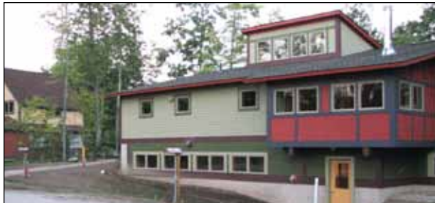
Common House at Rocky Hill Cohousing designed by Bruce Coldham.
